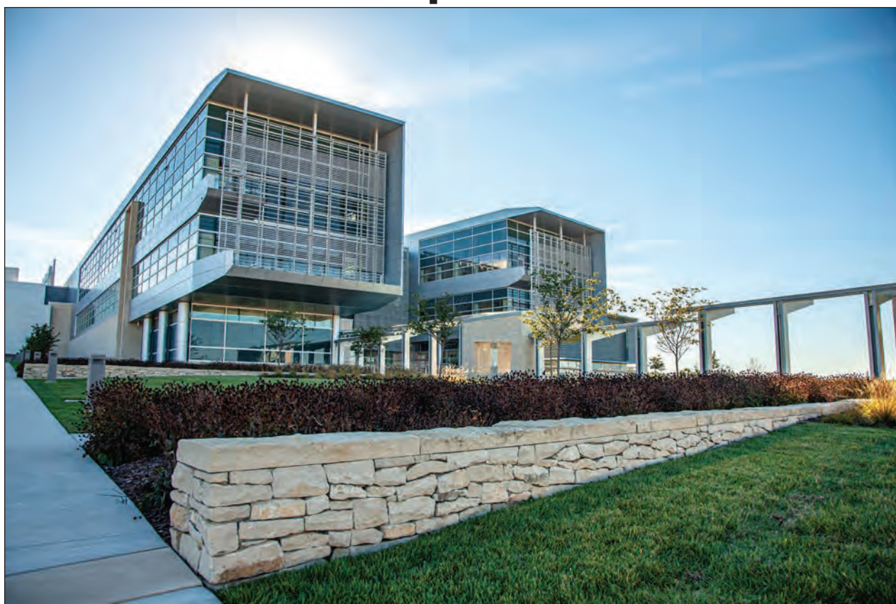
The construction and commissioning phase has been completed for the National Bio and Agro-Defense Facility (NBAF) in Manhattan, and it has now moved into a phase known as the operational endurance period, which will test and validate building systems before NBAF is transferred from DHS to USDA. Courtesy photo
