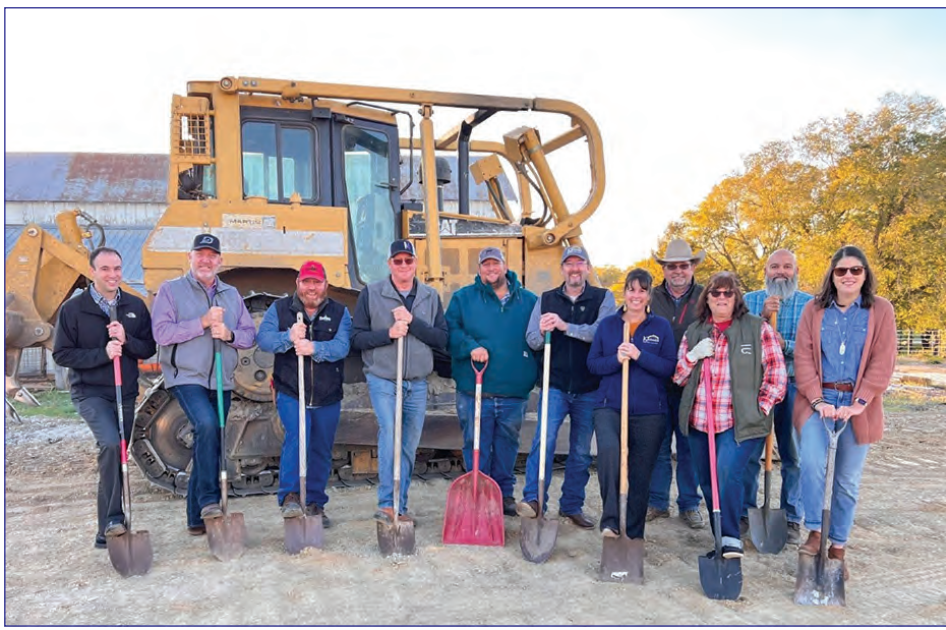
The Pottawatomie County Fairboard recently broke ground on a new multipurpose building that will be used by livestock projects during the fair and provide a larger more functional space for events throughout the rest of the year.
