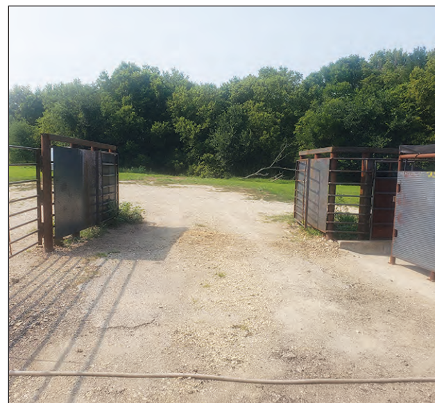
A pull-through area for unloading keeps customers from having to back up their trucks and trailers.
