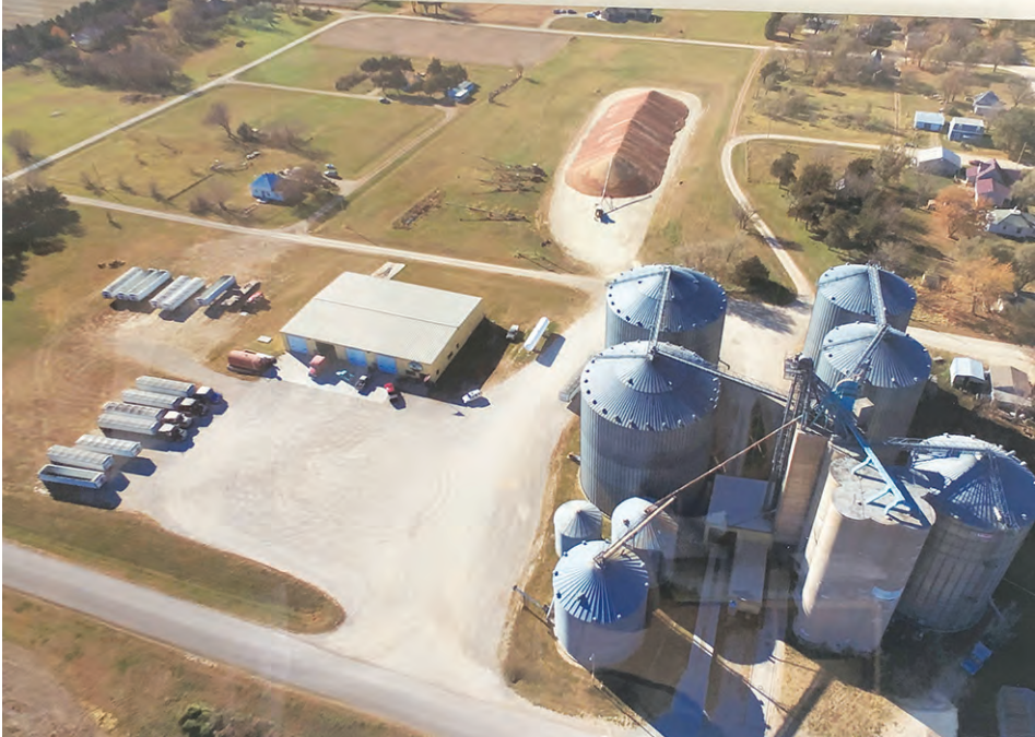
A more recent aerial shot shows the expansion of Lippert Grain Company in Green.
