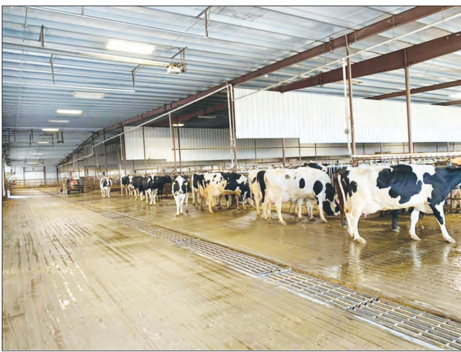
The first half of the cross-vent barn was built in 2016 and the second half finished in 2018. It gives the cows room to eat, sleep and roam around in a comfortable, climate-controlled environment.
