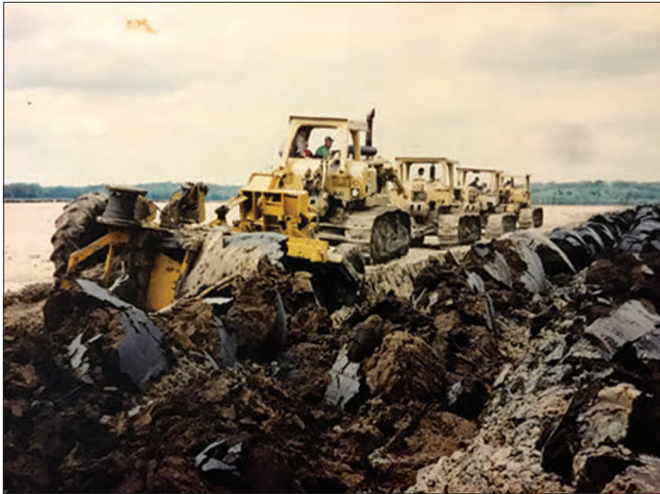
The Post plow, pulled by four bulldozers, mixed sand left by floodwaters with soil to restore farmland.
