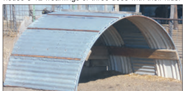
This is a water tank shed. An old metal bed frame was used for the back wall. It is recommended to double the spacing between the two arches of the tank.
