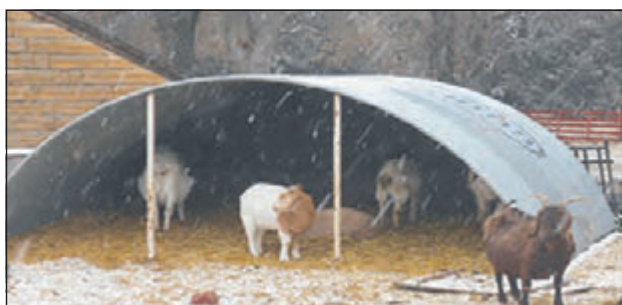
A grain bin was used to build this shed on skids. Two-thirds of the front can be covered to keep the wind out during the winter or it can be used open as in the photo. These are easy to clean out and can be moved with a tractor.
