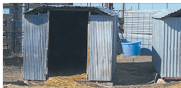
Stock rack sheds built on metal skids are heavy enough to not blow away in a storm and are easy to move with a tractor to clean old bedding. They can house 8-12 weanlings or three does with their kids.
