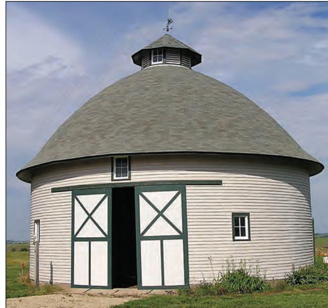
This 1918 round barn southwest of Marysville was sold as a kit by Sears Roebuck. It is the only Sears round barn in Kansas, owned by Rick and Carol Wright, who take great care of this piece of history. This early model has curved doors; later ones were flat.
