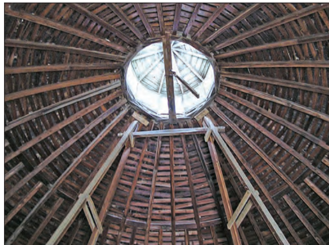
This photo offers an inside view of the barn's roof.
