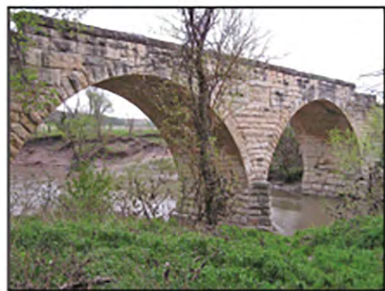
Limestone Arch Bridge, Clements
