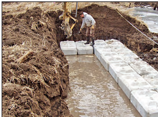
A Block Chute Structure at the Luedder farm was constructed to solve the problem of "head cutting" where a waterway meets the stream.
