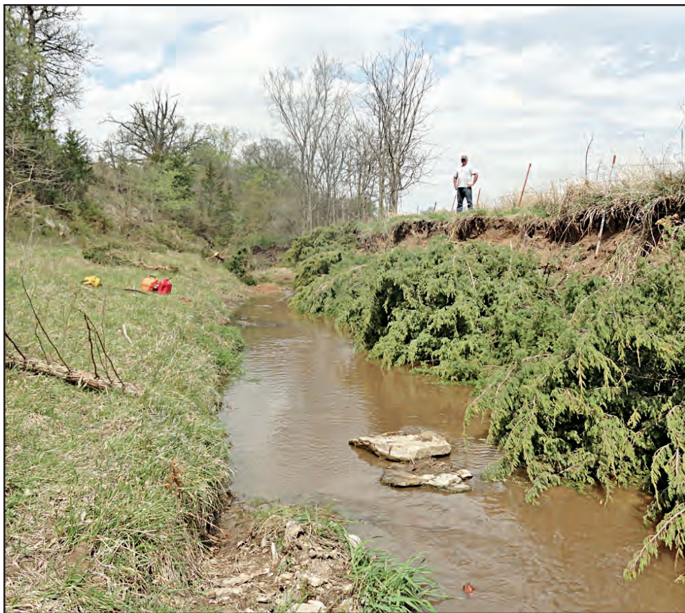
A cedar revetment project along Elm Creek in Marshall County helped stop erosion on 90 feet of its streambank.
