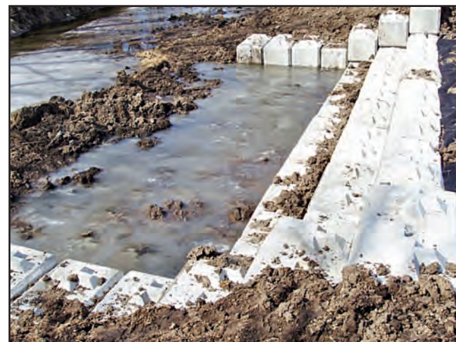
Starting at stream level, the blocks create a wide pad where flowing water enters the stream. They are then stacked in progressive stair-steps.
