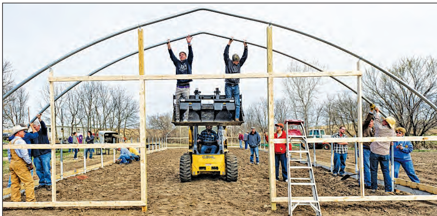
Bows were maneuvered into position with the use of a skid loader and helping hands.
