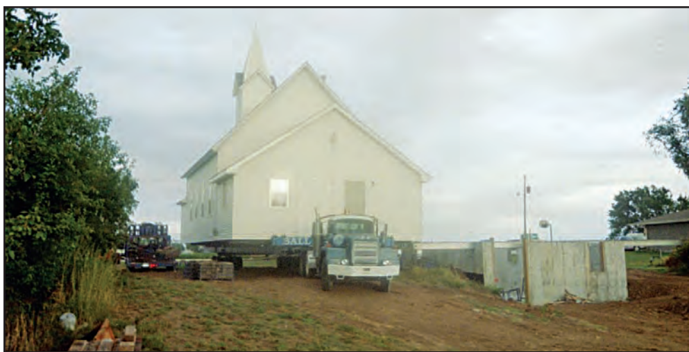
A deteriorating basement forced the move of the Rose Valley United Methodist Church in Downs. The church was moved thirty feet sideways, then replaced upon a newly constructed basement.
