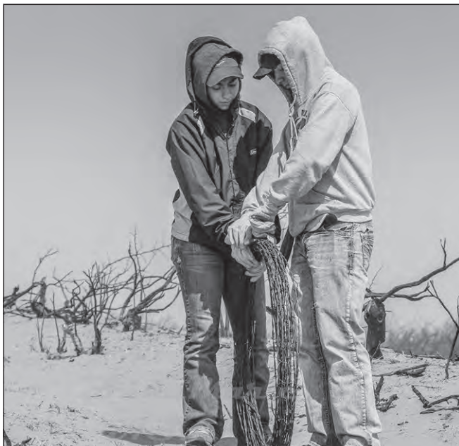
Pulling out damaged fencing and laying wire were the activities that filled the days of these young people.
