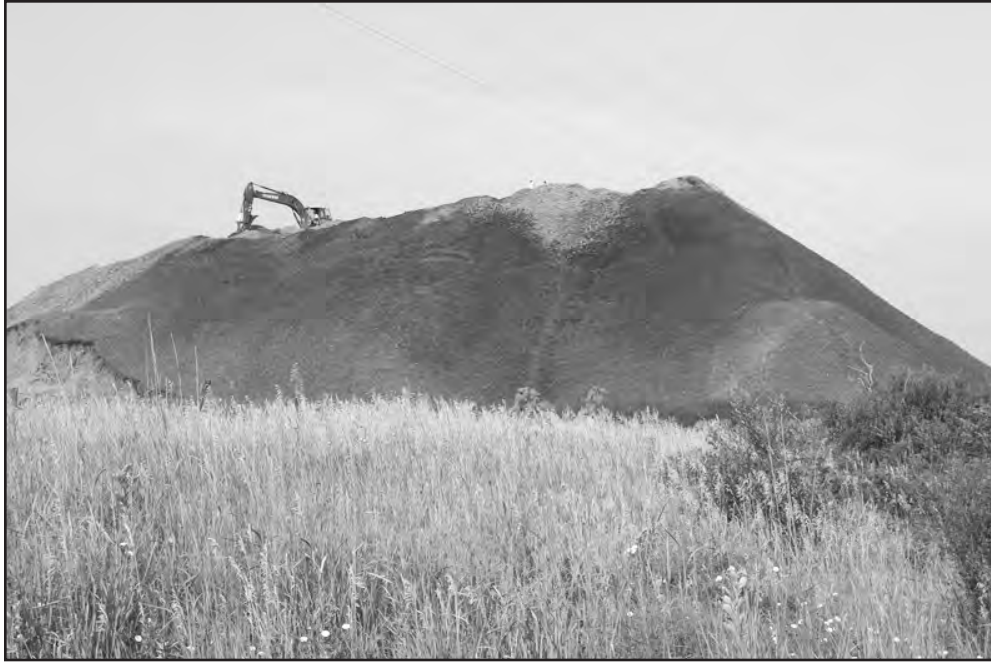
An excavator digs through the 75-foot pile of corn cobs looking for any hot spots.
