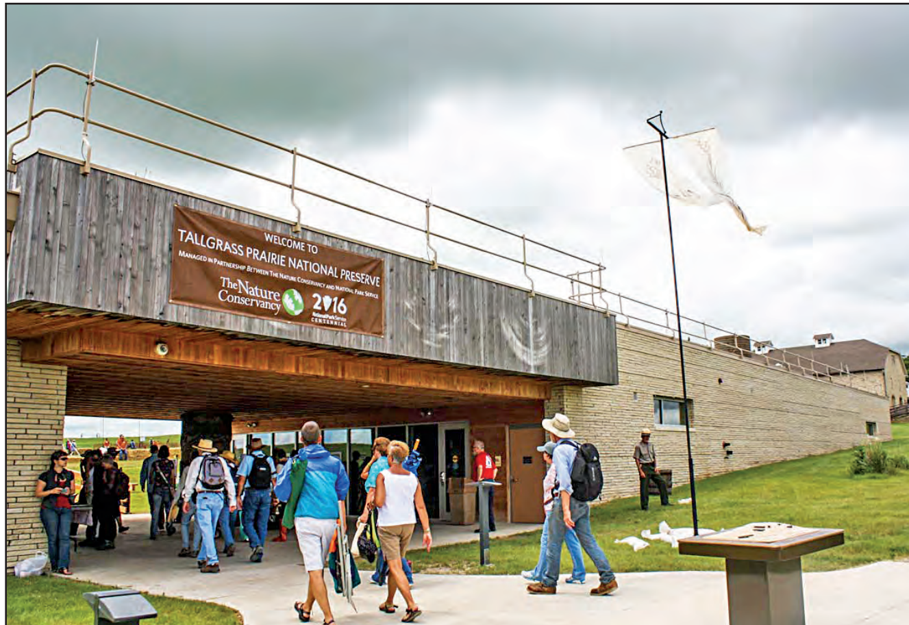
The new visitor center at the Tallgrass Prairie National Preserve is designed to foster an understanding of the importance of the last remnant of tallgrass prairie found mostly in the Kansas Flint Hills.
