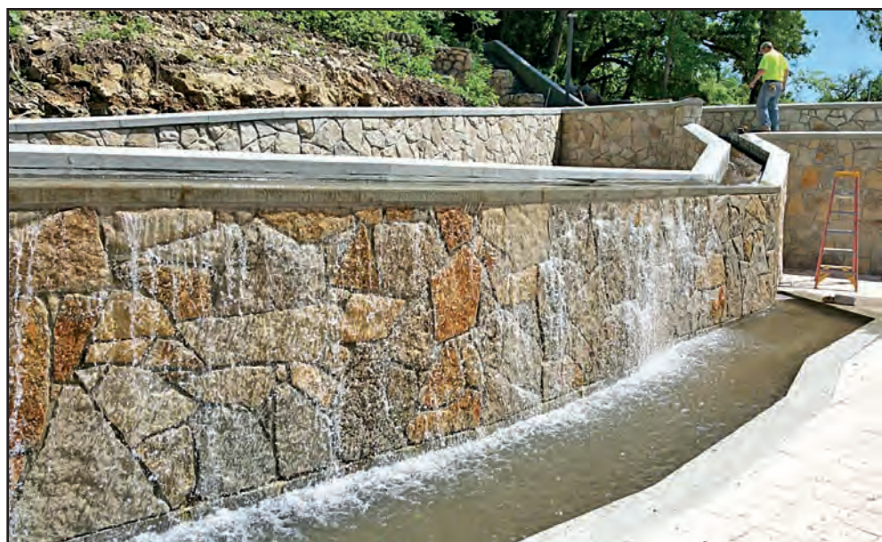
Water cascades over the new spring wall.
