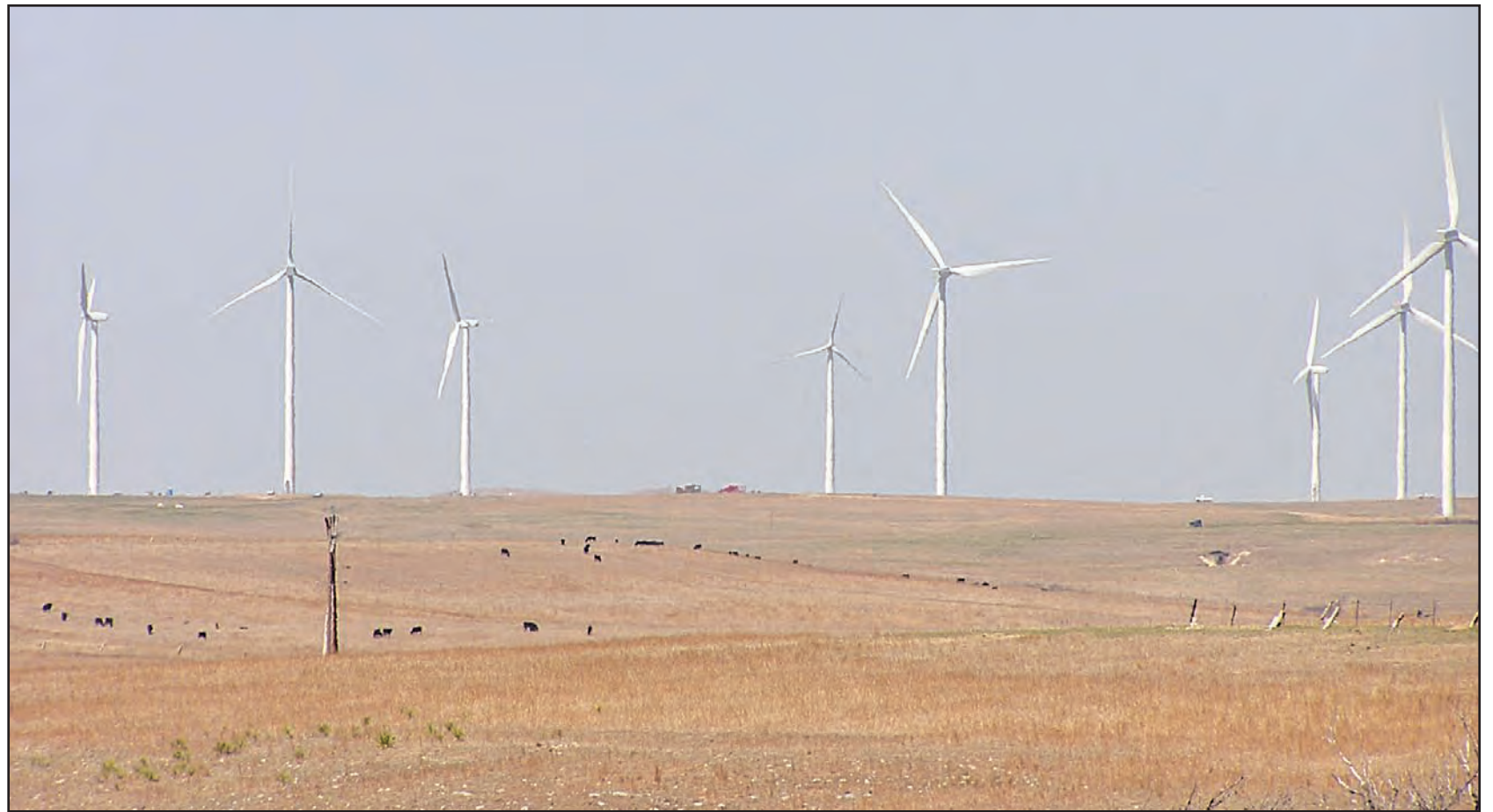
It is a blend of old and new that drivers along I-70 will find just west of Salina in Ellsworth and Lincoln counties. The new Smoky Hills Wind Farm is in various stages of construction, including some of the giant turbines that are now operational. A herd of cattle contentedly graze the rolling hills below, seemingly unfazed by the new windmills that dwarf the old-fashioned water windmill.
